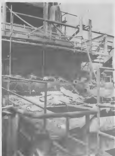
Boiler no. 10 at Powerhouse no. 1, the oldest boiler at Lago dated back to 1939, is presently being dismantled in connection with the Utilities Modernization Project.
